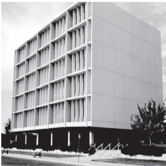
Figure 1: Imperial Country Services Building, El Centro, California (U.S. Geologic Survey)
